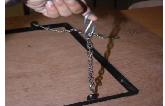
Suspender chains attached and ready for ceiling suspension
