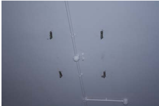
Hooks bolted into the ceiling at the site for suspending entire assembly
