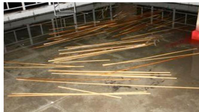
Fig45: the bamboo strips soaked in water before bending.
