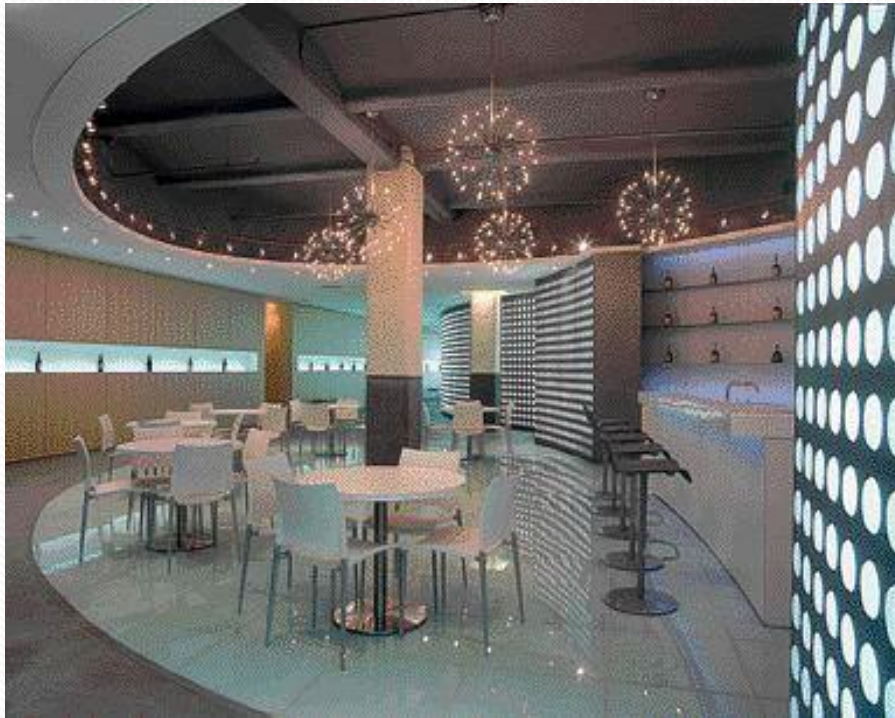
To Ensure An Error-Free Installation, the 250-Foot-Long Wall Was Constructed Using a Template Affixed to the Rough Concrete Floor
