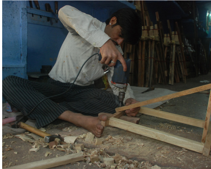
Finally fixing the other end of the piece to the top portion of the structure.
