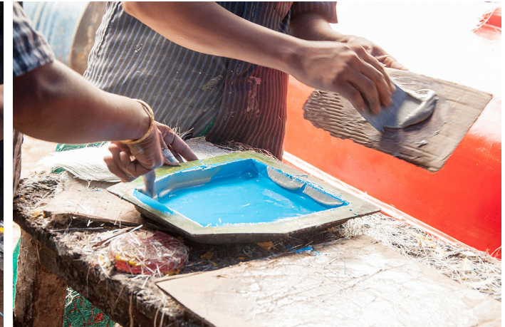
Second coat of the resin solution is applied.
