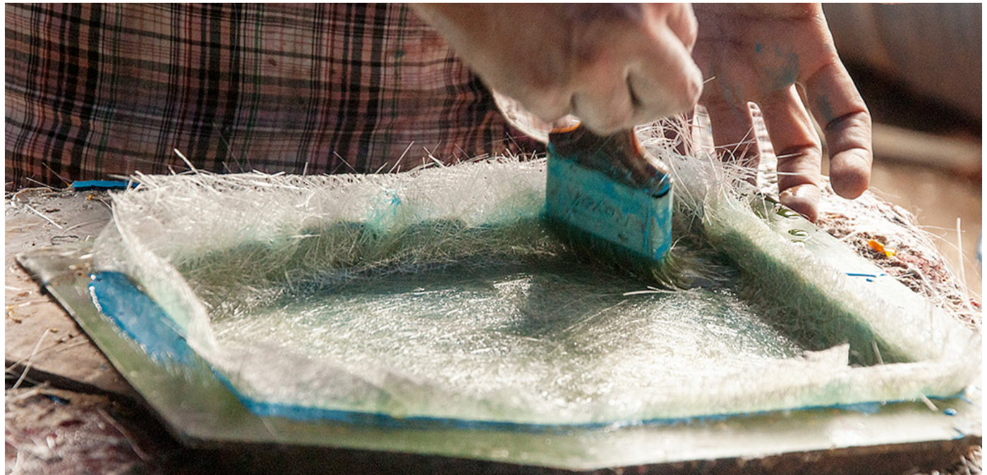
Resin is being applied on the fiberglass mat to remove the air bubble.
