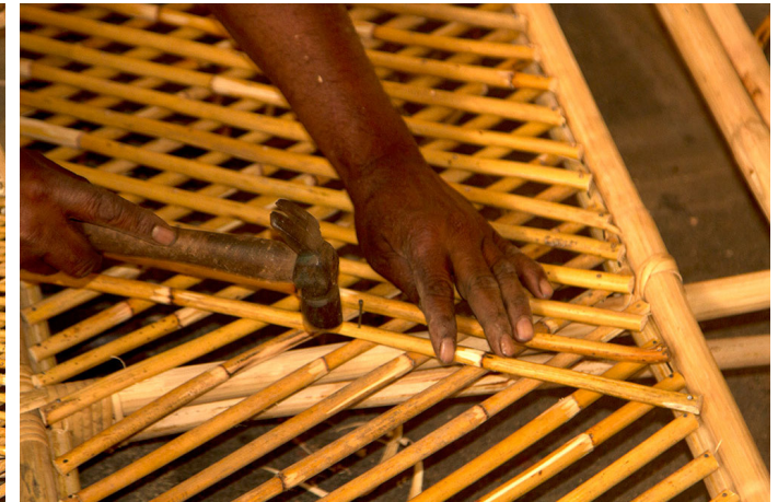
Metal nails are used to fasten each pieces in diagonal manner.
