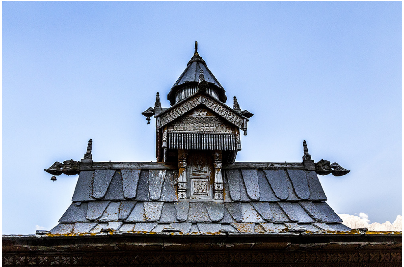
Roof of slates.
