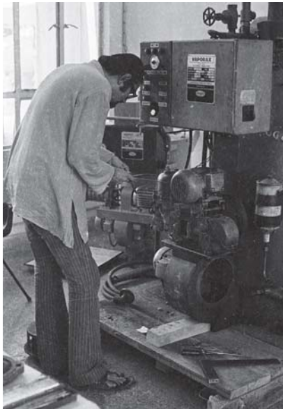
35. Prof Athvankar working on the Wansons boiler
