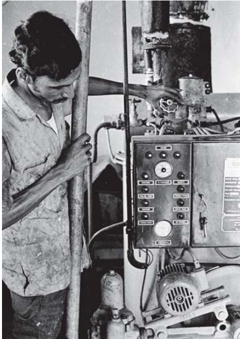
33. The old Wansons boiler
