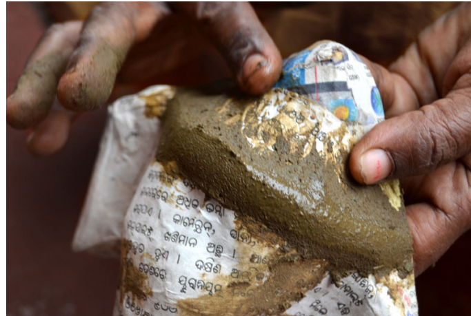
Cowdung being coated on the layer of paper.
