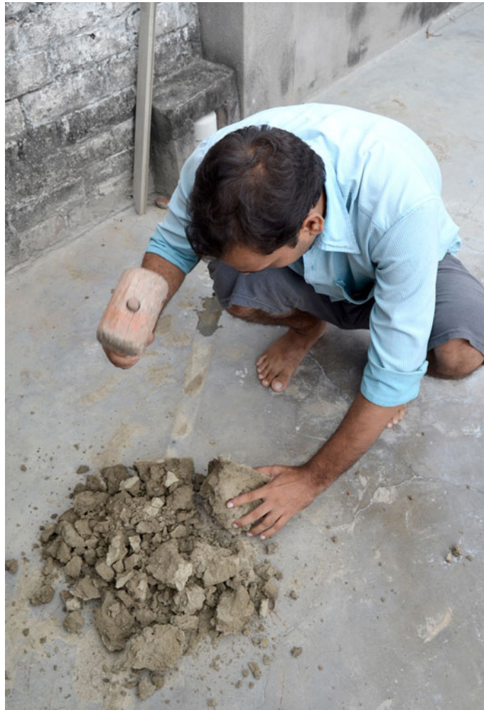
Pieces of solid clay being broken down.
