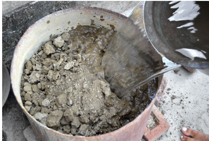
Clay pieces being mixed with water.
