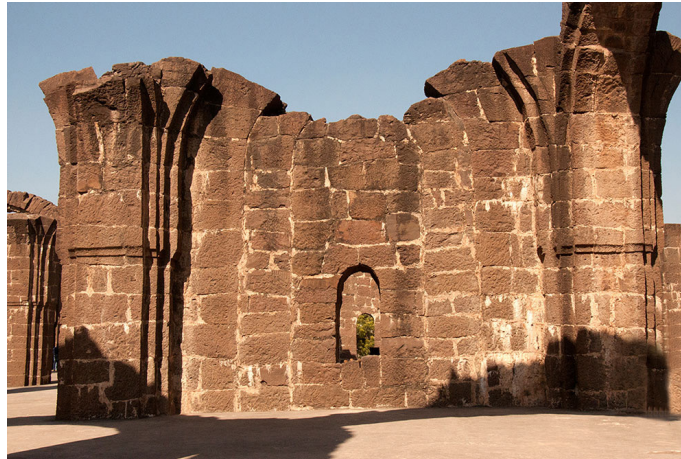
Solid wall in the form of concentric arches.
