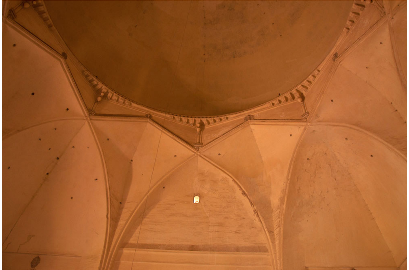
Dome with intersecting arches.
