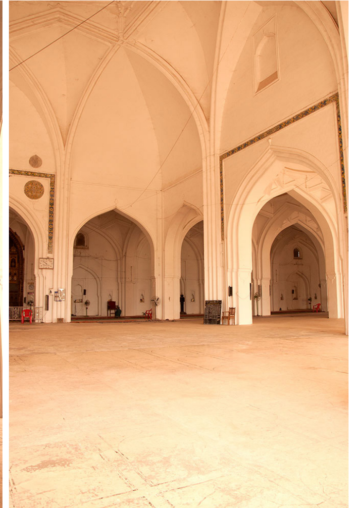
The interior of the sanctuary is a large hall 208' X 107', divided into five aisles by arches on large masonry piers.
