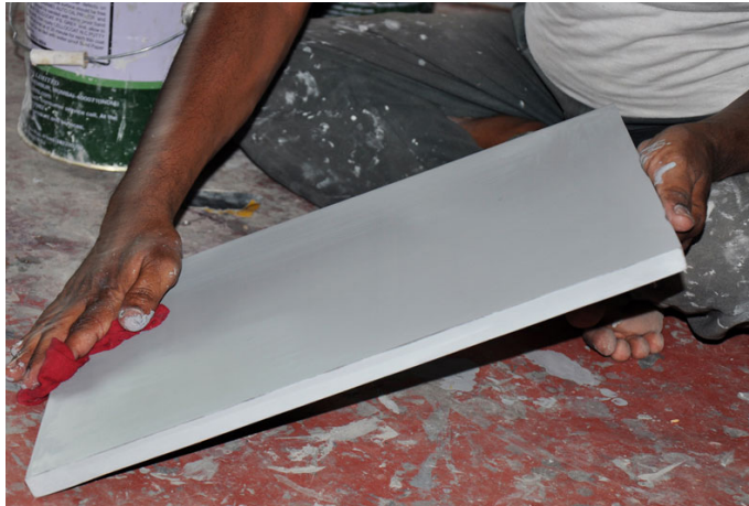
After coating, the surface is smoothened.
