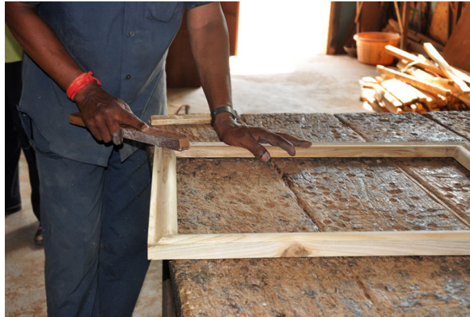
The frame is smoothened before painting to obtain smooth surface.
