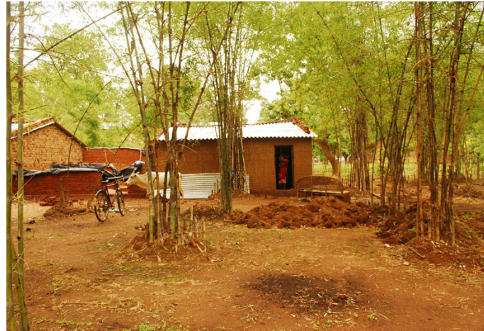
Newly built cottages for craftsmen.
