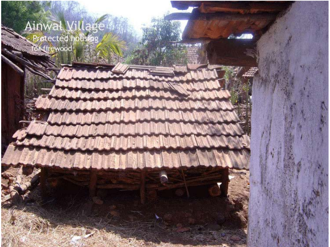
Protected housing for the firewood.
