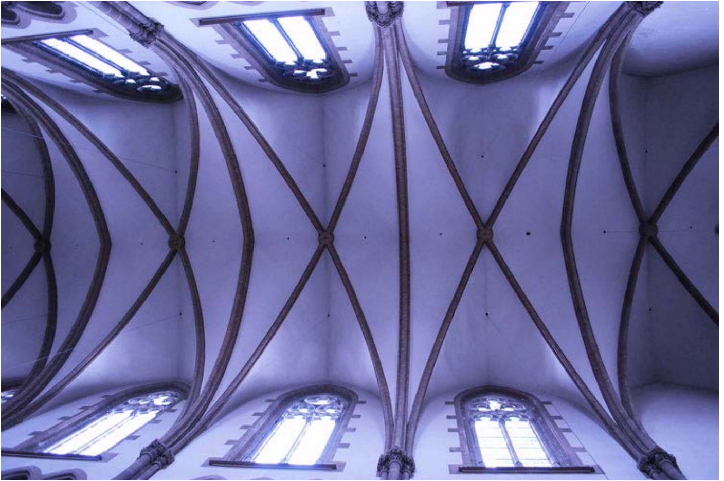
Ceiling of a church featuring a play of lights and shadows.
