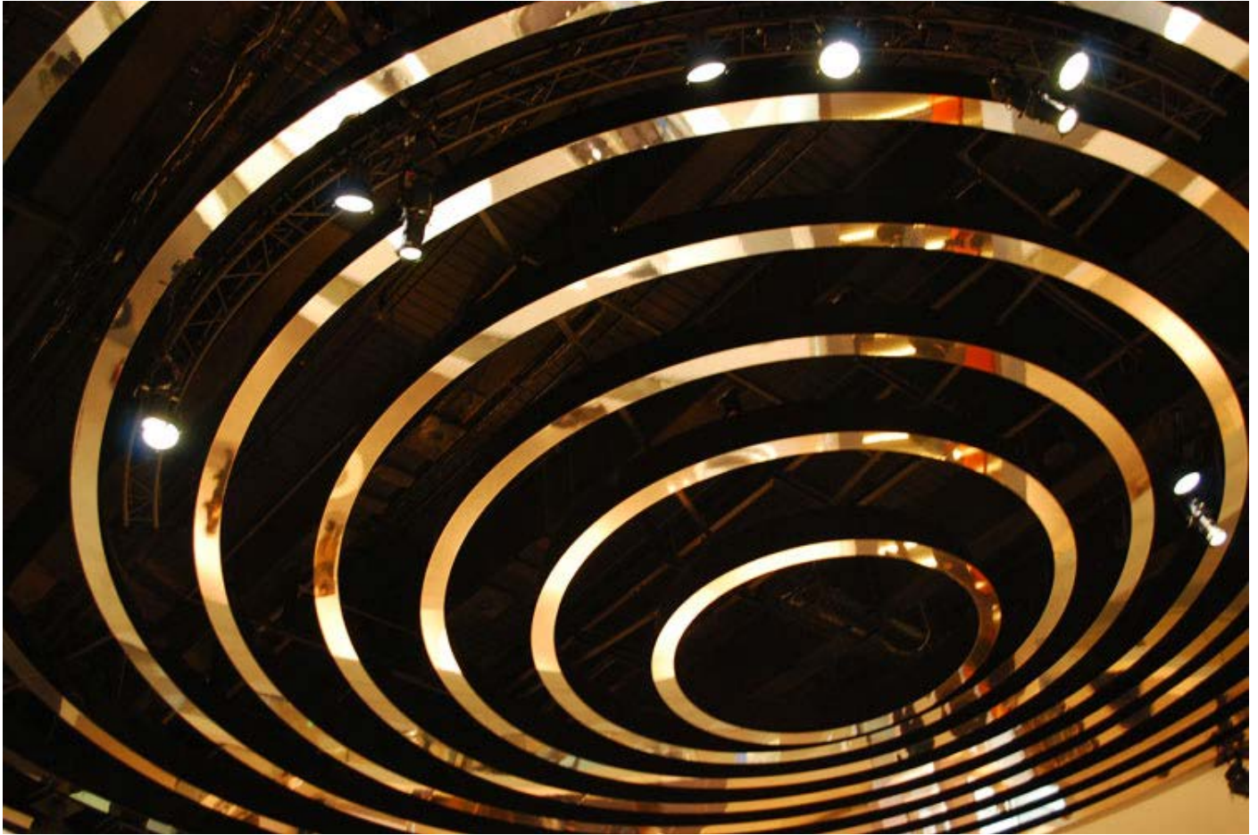
Ceiling of a public museum appears to drop in due to the radially reflective tracks.
