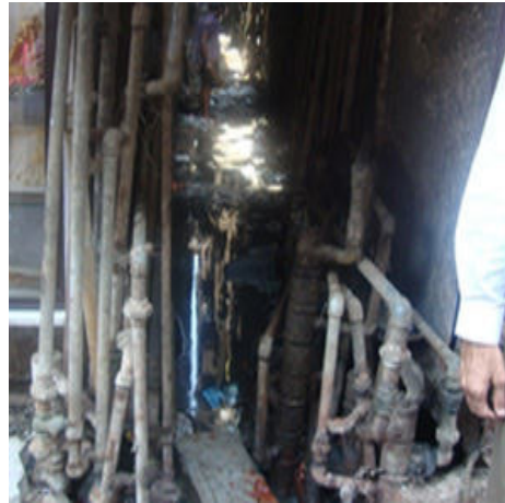
Fig 17: Narrow gullies with water pipes
