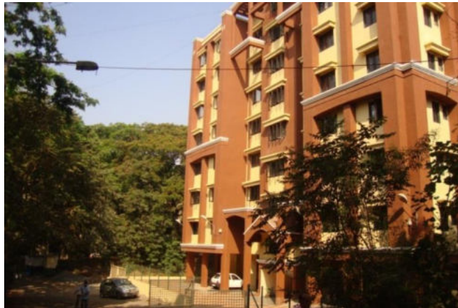
Fig no. 28 Residential building inside IITB
