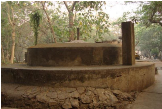
Fig. 54 Bio gas plant at IITB Staff canteen
