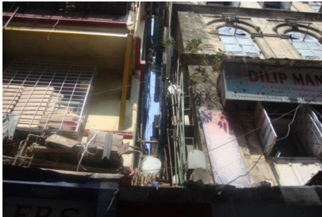
Fig 21. A Little gap between buildings called "Gully"
