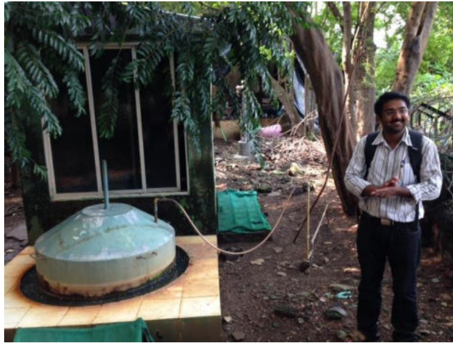
Fig 32 TISS Biogas plant
