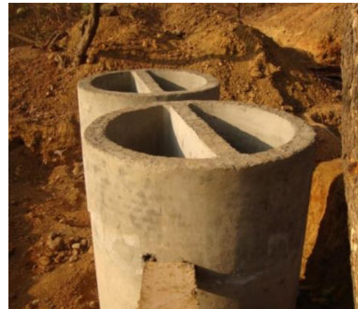
Fig. 38 bio gas plant at IIT Bombay.
