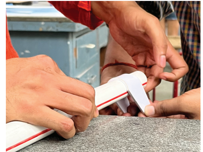
The bracket cut from styrene sheets were bent on the pipes using heat gun.
