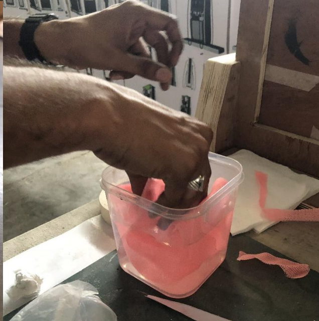
• FRP Bandage coated with Resin.
