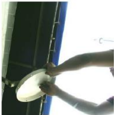
central plate was drilled at the center of the canopy.
