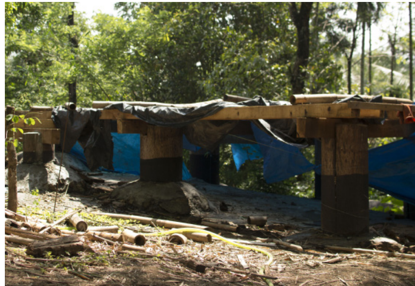
Fig.36: Palm and concrete structure for base construction
