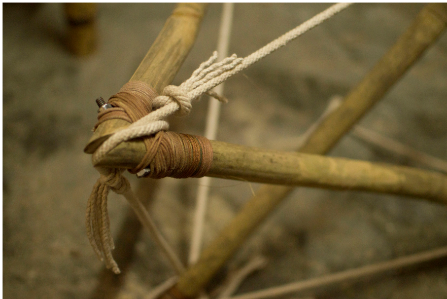
Fig.39: Clockwise from top-left 1. 7-shaped struts, 2. tensegrity structure 3. Cotton rope as tension member, 4.Join area of struts; source : Author
