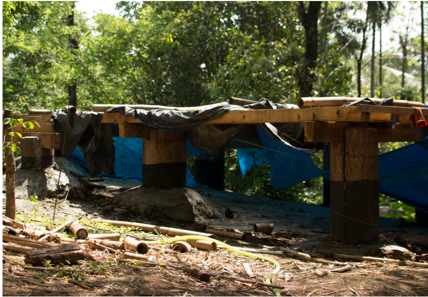
Fig.27: Palm and concrete base for construction; source: Author
