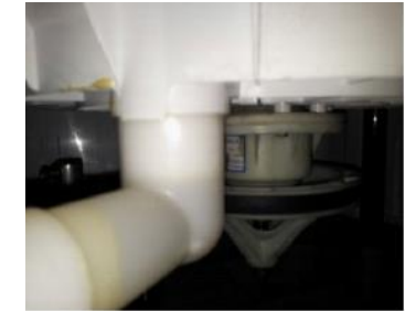
Outlet pipe fixed to washer
