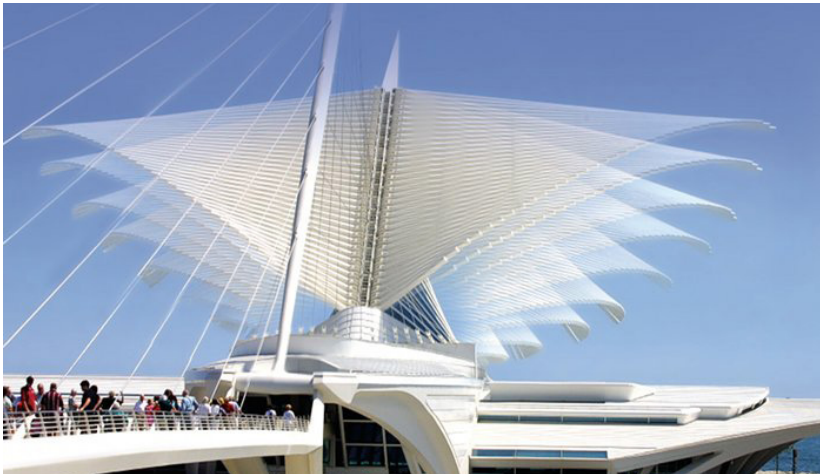
Fig 37. Transforming roof structure at the Milwaukee Art Museum by Calatrava
