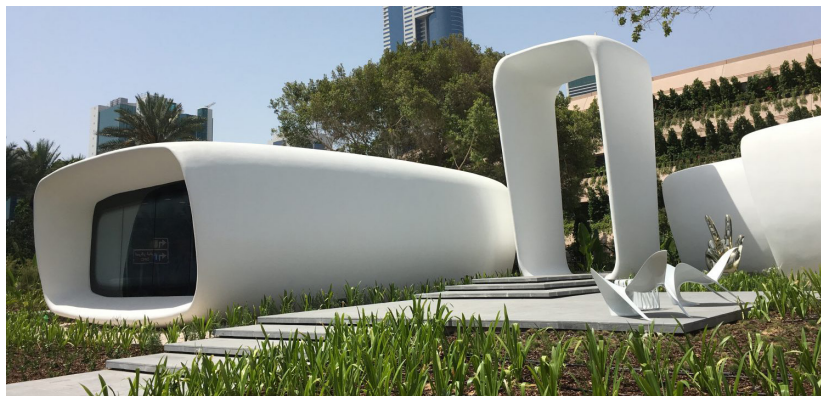
Fig 47. 3D printed office building in Dubai, UAE
