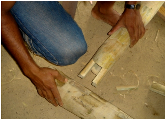
Fig. 3.20 Tenon and Mortise joint in Bamboo
