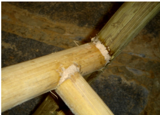
Fig. 3.22 Gaps filled with Sawdust and Fevicol
