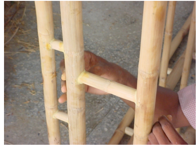
Bamboo mixed with Mseal used to fill gaps
