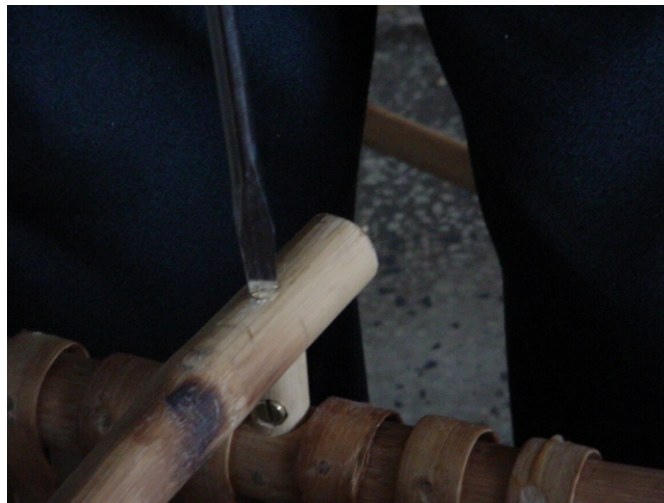
Brass nut and bolt used to hold the joint
