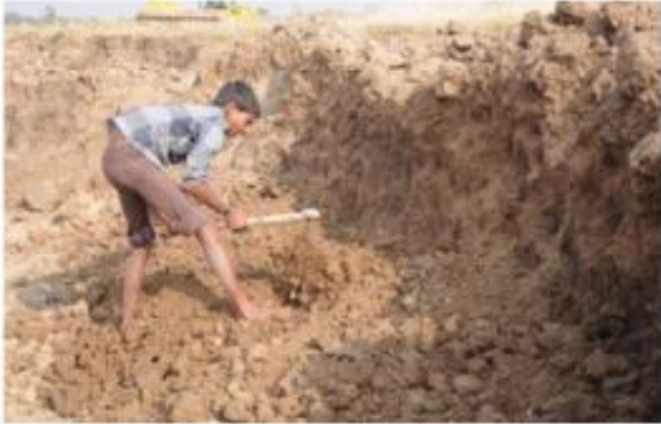
Fig 15 : Breaking larger soil lumps into smaller fragments
