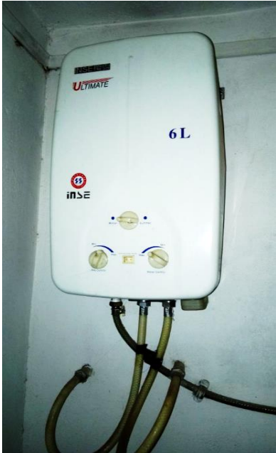
FIGURE-11 Water heater mounted at top corner of bathroom with almost not accessible to operator for people with shorter height.
