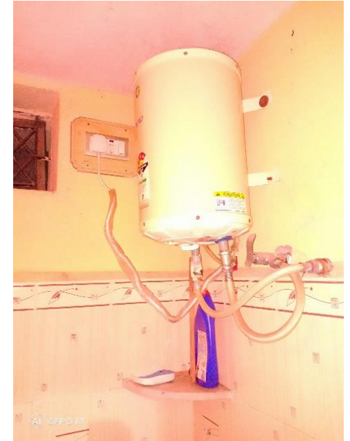
FIGURE-14 Water heater mounted inside the bathroom in the corner at with all pipes obstructing space of users to access.
