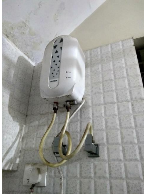
FIGURE-12 Water heater mounted inside the bathroom in the corner at high height of 8.5 feet.
