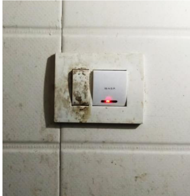
FIGURE-13 Switch of the wall concealed unit gets dirty in as it is located inside the bathroom.
