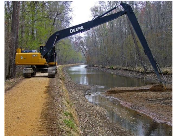
Fig 2(Desilting Process)- http://budcline.aminus3.com/image/2012-03-12.html
