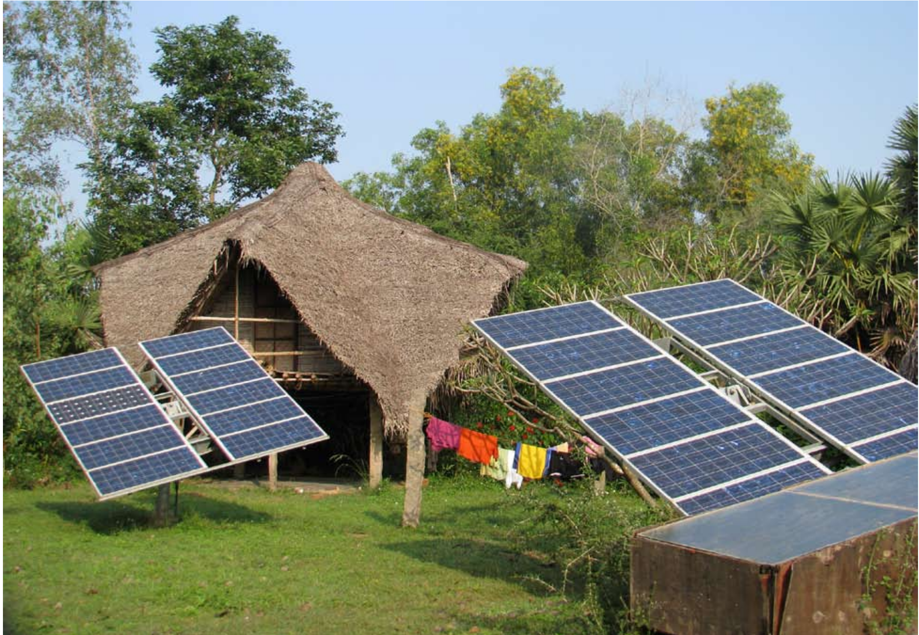
Sustainable living practices at Buddha Garden: The solar panels getting charged with the sun energy in the daytime while the agriculture experts till the land and sow seeds with the help of volunteers
