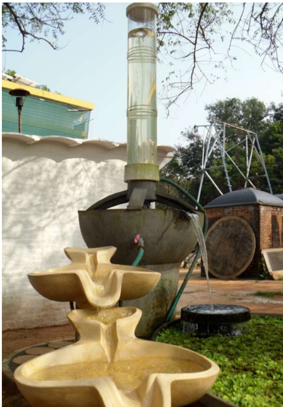
Waste water treatment setup and 'green' plants outside Satprem's office
