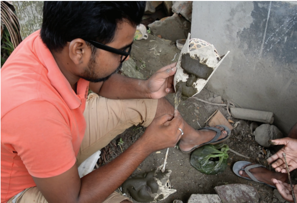
The mixture is applied using a bamboo or metal spatula
