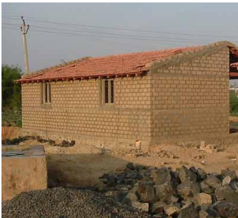
Figure 3.10 Fly ash brick wall construction
