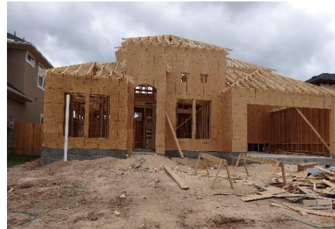
Figure 3.24. House made timber frame construction method
