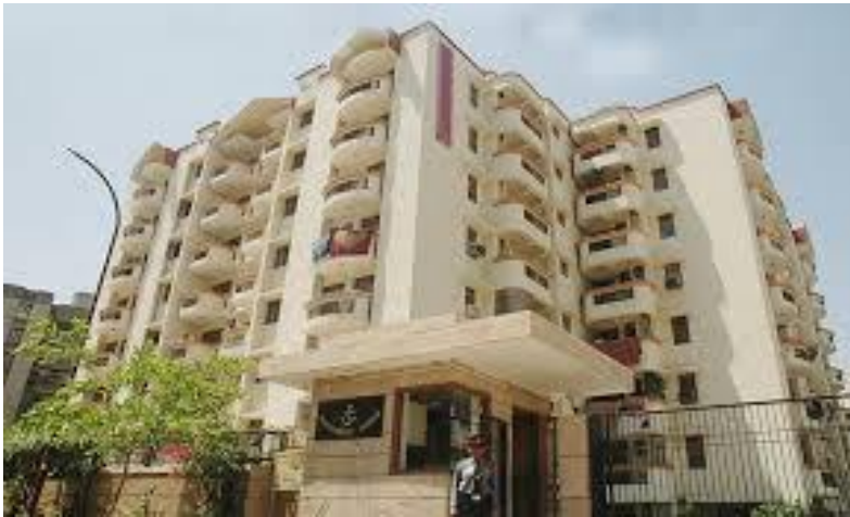
Figure 3.1 Building construction in metro cities
