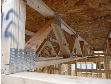
Figure 3.28 Beam and its joining plate
