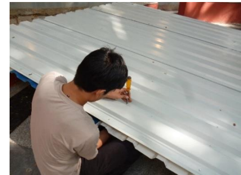
Joining by nut bolt
