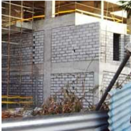
Figure 3.9 Concrete brick wall construction
