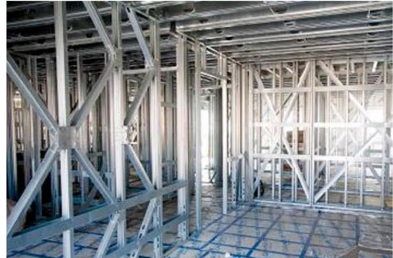
Figure 3.32 Light weight steel frame construction
