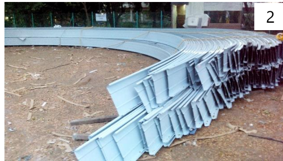
Roofing Sheet – Bent in a curve (Bending machine transported onsite)
