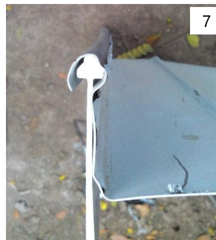
Sheet with end 1 fitted over the plug
