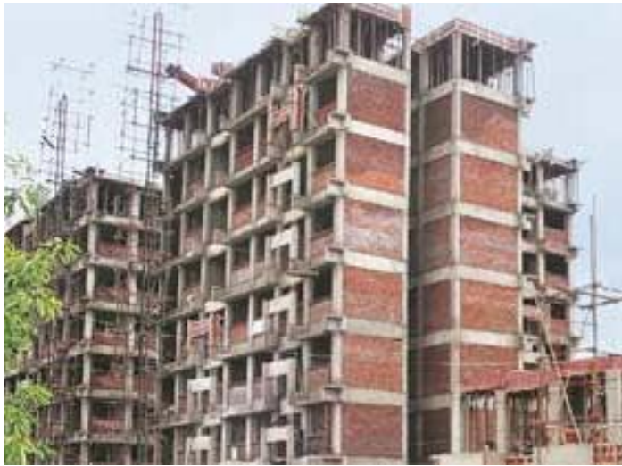
Figure 3.4. Building construction using concrete and red clay brick
