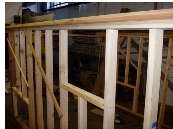
Figure 3.34 Caravan Wall Construction
