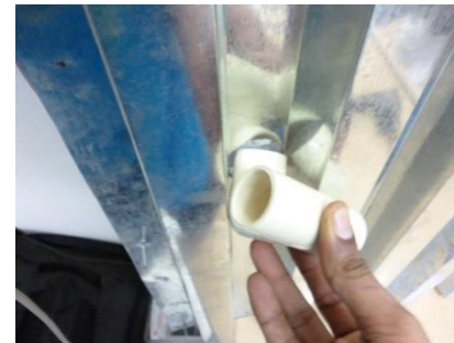
Image 8.3 insertion of T joint into the corrugated sheet
