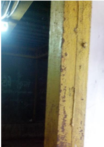
Fig3.22. Column made of 2 'C' joining together
