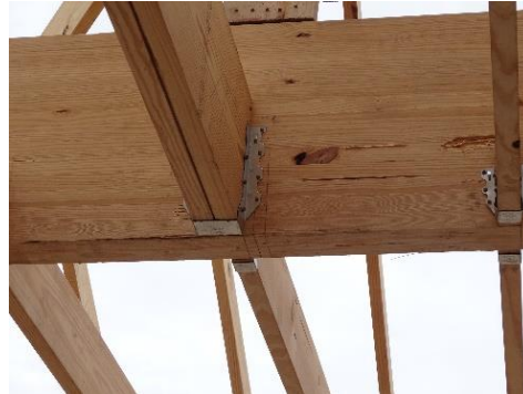
Figure 3.29. Joint for beam support
