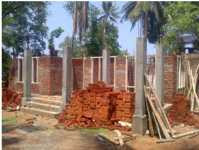
Figure 3.5. ground +1 floor house construction
