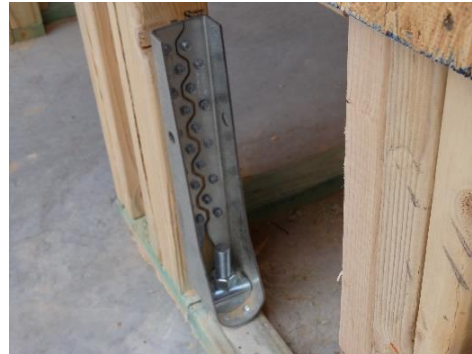
Figure 3.31 detail for fixing stud with floor
