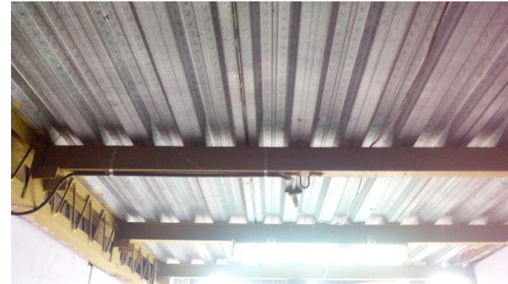
Figure 3.20. slab construction using corrugated sheets
