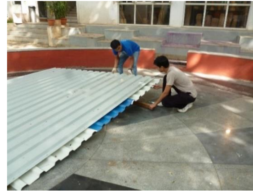
support for drilling
