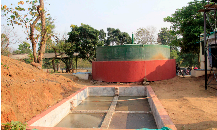
Biogas plant based on BARC technology. Capacity - 2 Tons per day.
