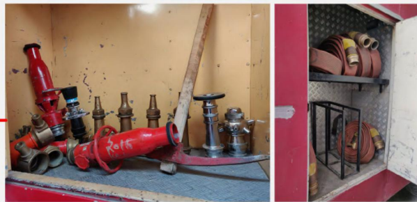
Storage area for hoses and different nozzle with coupling for hose attachments
