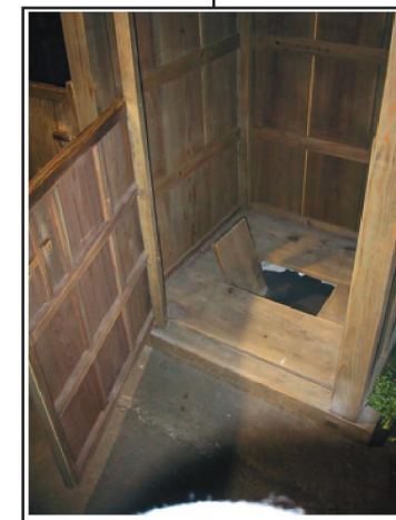
Fig.25. Japanese pit toilets
