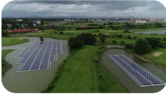
Cochin International Airport Limited (CIAL) major floating solar power plant
