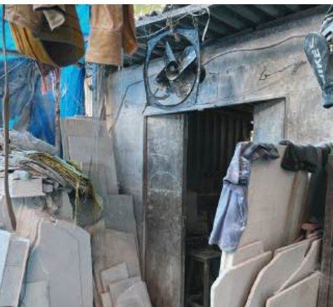
Fig 12.5: Exhaust Fan Installation
