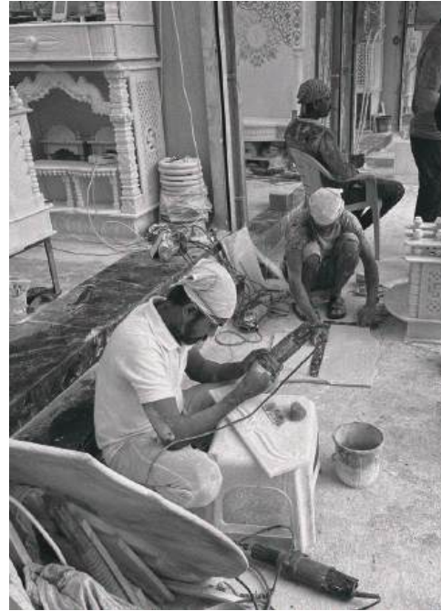
Fig 13.2: Encroachment Outside Workshop
