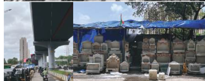
Fig 1.3: Metro Station, Malad W
