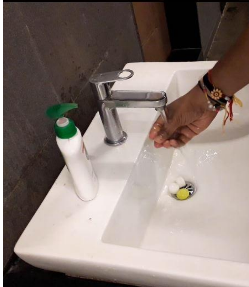
Fig: Hand washing under Faucet-1 (urban setting), Aerated water outlet- feeling of more water but time-consuming to wash, due to lower pressure compared to jet flow.
