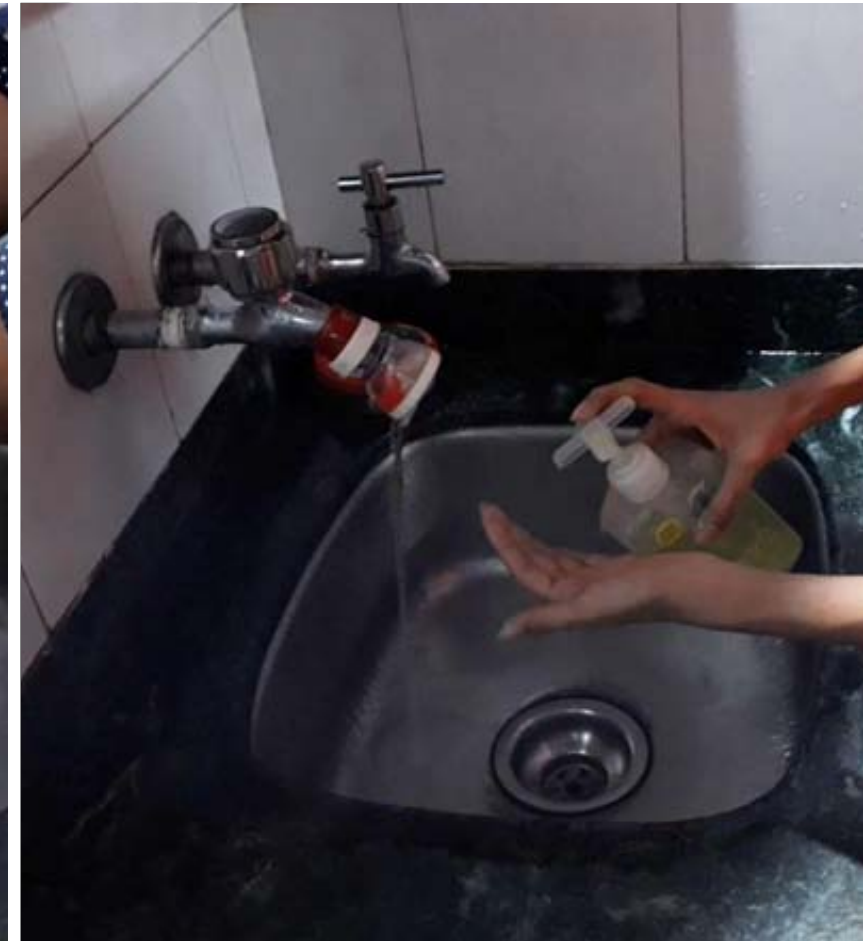
Fig: Washing hands under Faucet-4 (rural setting), Faucet is left ON during the whole process of washing hands, but the water output is kept low throughout.
