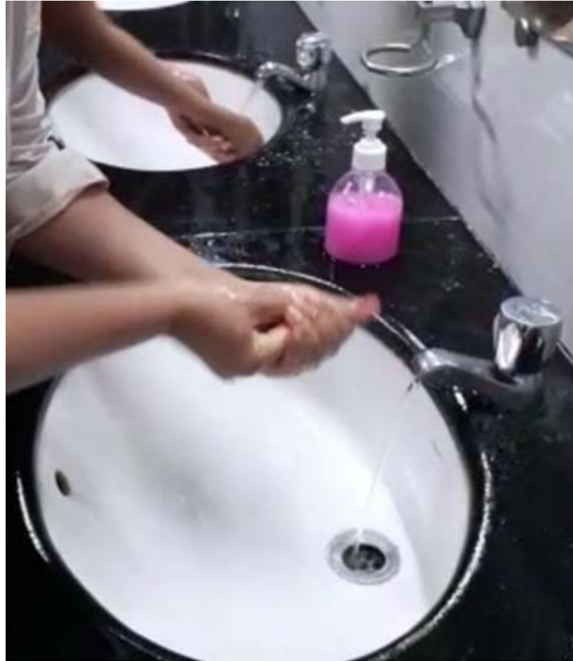
Fig: Hand washing under Faucet-3 (urban setting) Difficult to operate knobs result in people leaving it ON throughout usage.
