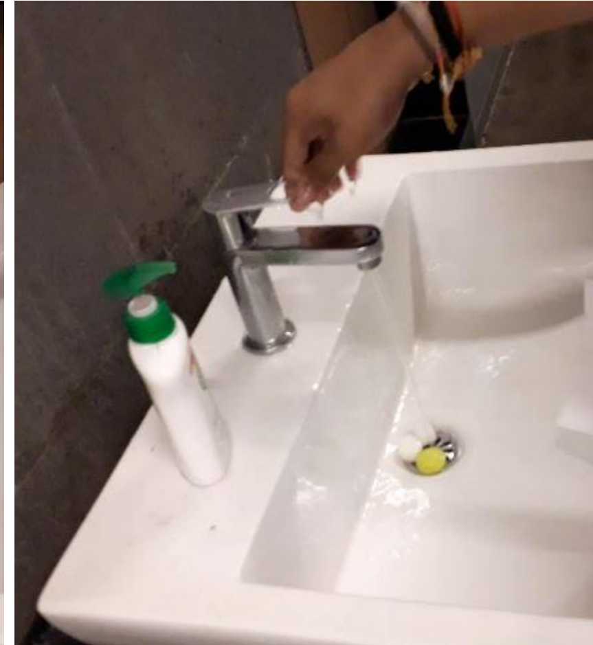
Fig: Washing hands under Faucet-1 (urban setting), Ease of operation, quicker ON/OFF functions
