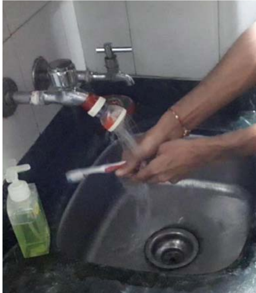
Fig: Hand washing under Faucet-3 (rural setting), Additional accessories fit onto the fitment to increase the spread of water outlet.
