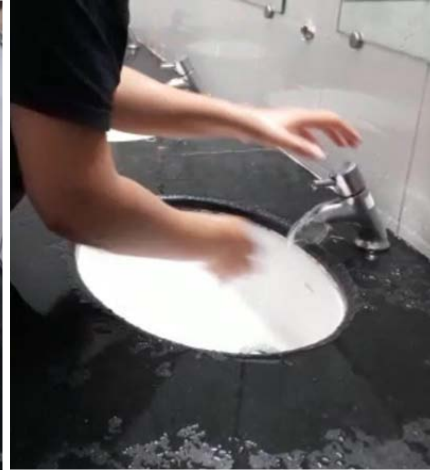
Fig: Washing hands under Faucet-4 (urban setting) Ease of usage due to the long, protruding knob.
