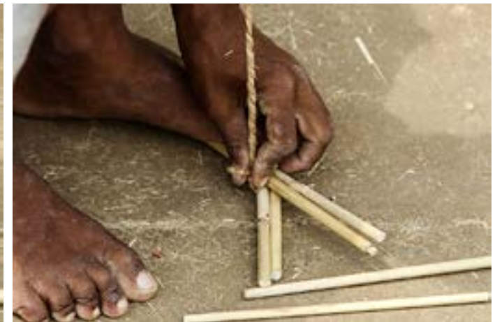
Bamboo sticks are tied together with bamboo twines.
