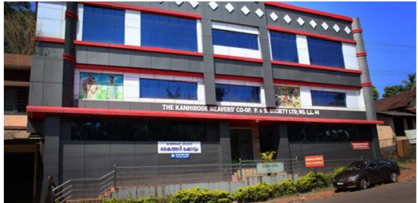
Weaving society office building.
