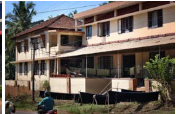
Weaving workshop building.
